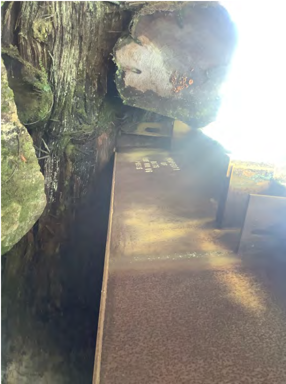
Left Bank Abutment when facing downstream
