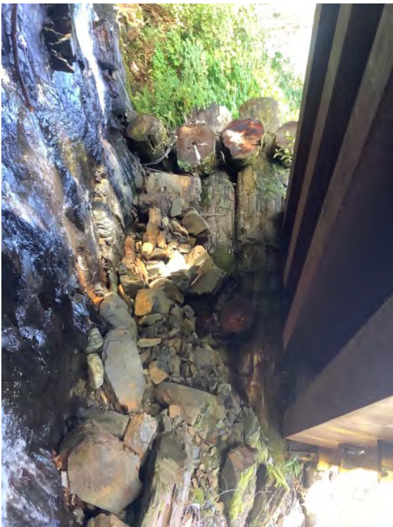
Right Bank Abutment when facing downstream
